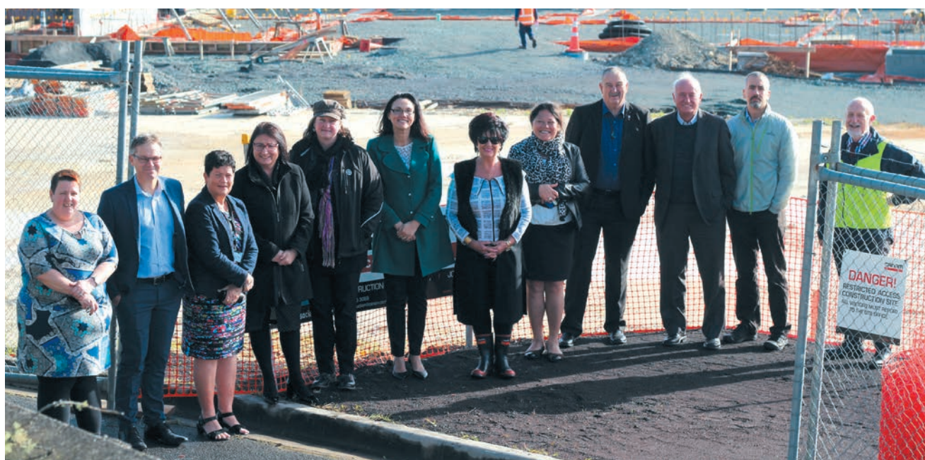
The Board at Bay of Islands Hospital Stage One building site checking on progress in October 2017.
